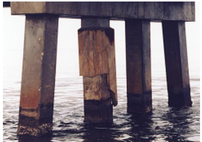
*Failure of a non-structural pile jacket.*
