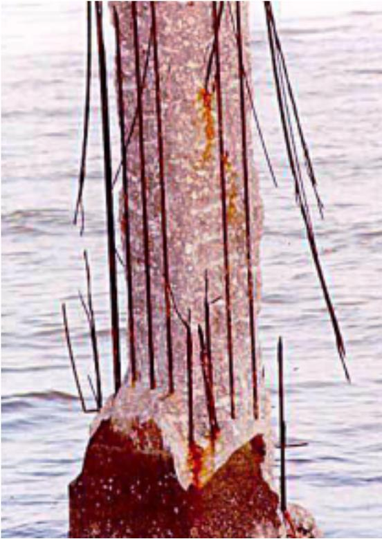
*A severely deteriorated pile which had previously been repaired with a fiberglass jacket.*
