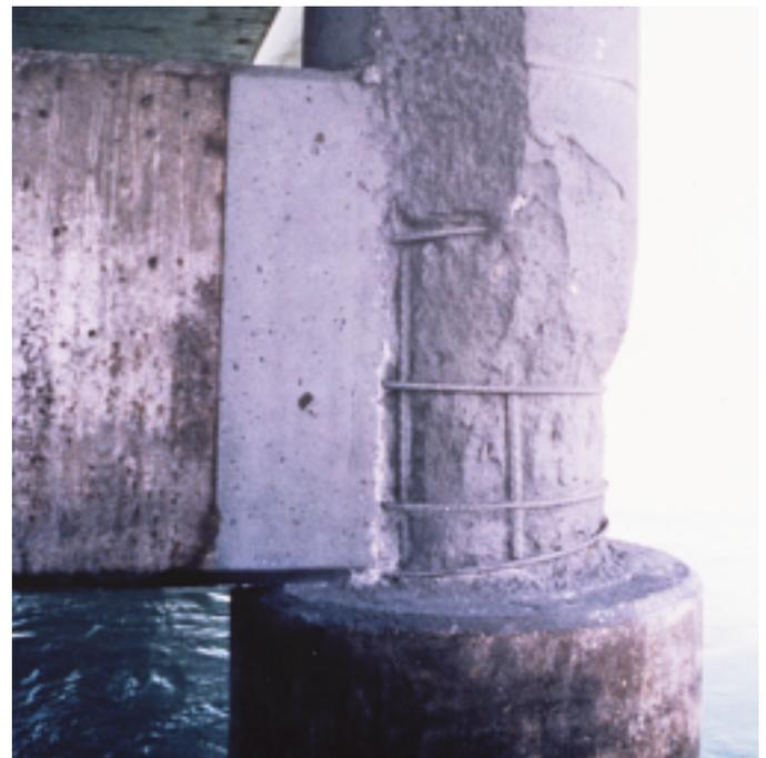
*A thin layer of zinc is applied directly to cleaned steel and adjacent concrete surfaces as part of the galvanic system.*
