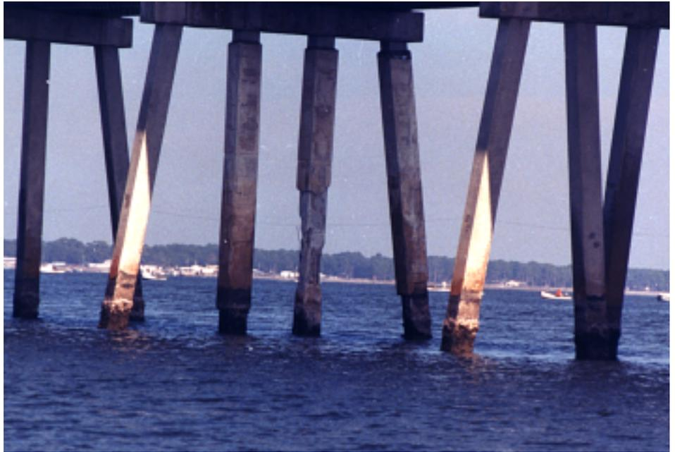
*One of the Bryant Patton Bridges in Florida displays a reinforced concrete pile with significant corrosion induced damage.*
