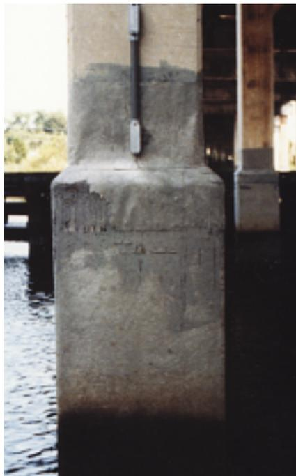
*The integral pile jacket system uses a fiberglass jacket supplied with the mesh anode.*
