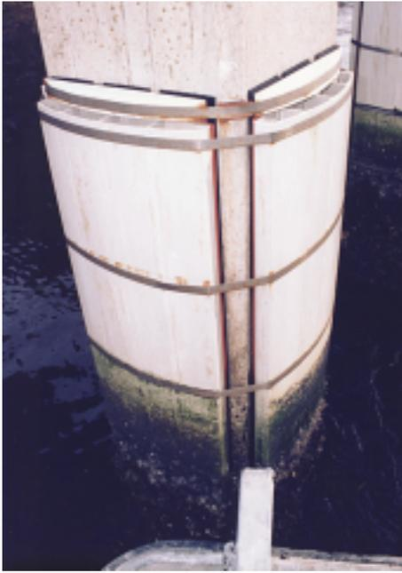
*This conductive rubber jacket system is protecting the tidal and splash zones of a bridge piling.*
