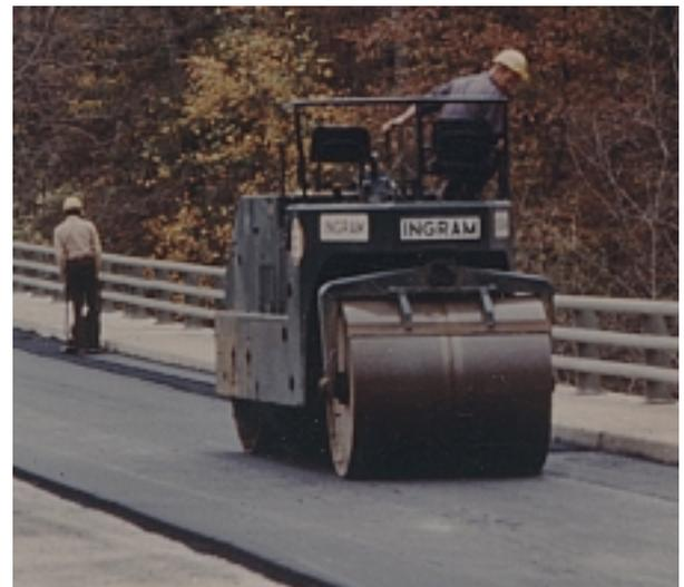
Figure 3. Workmen install Coke asphalt CP system.
