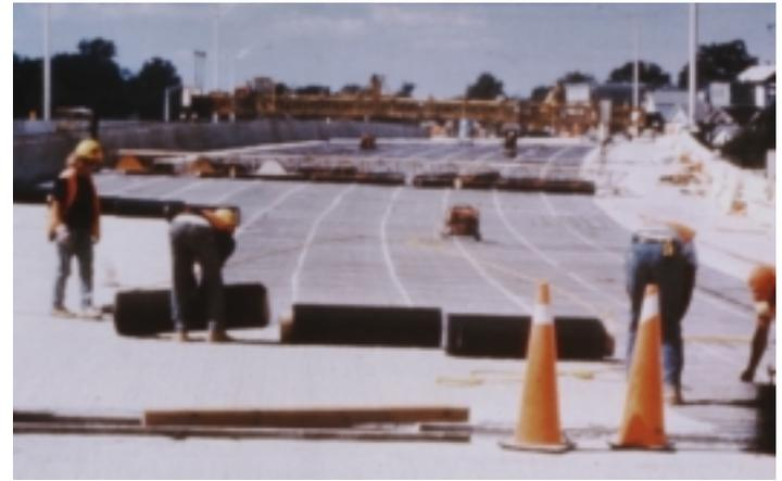
Figure 4. Mounded conductive polymer CP system.
