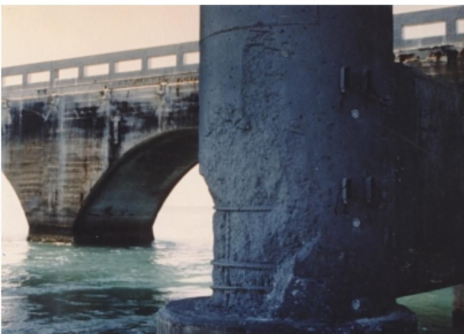
Figure 11. Flame sprayed zinc CP system which provides sacrificial CP
