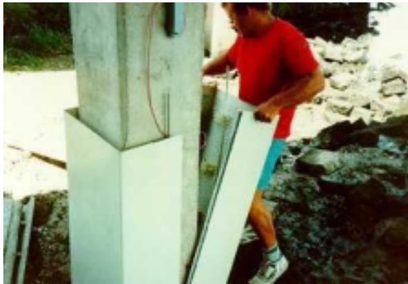
Figure 9 (above) and Figure 10 (right). Integral pile jacket CP system.
